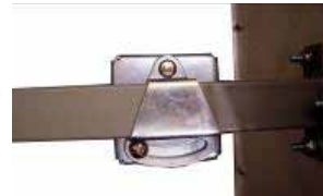
Bracket mounted for Down-Tilt
